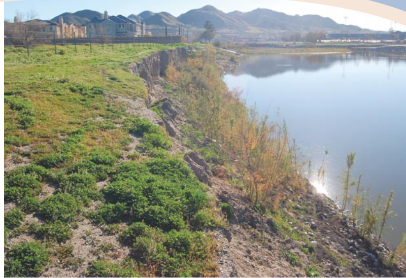
A damaged slope resulting from sedimentation and changing hydraulics in the Inlet Channel.
