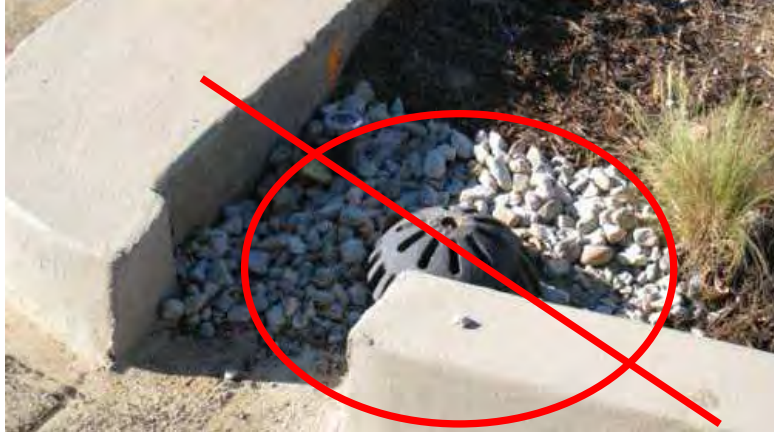
Figure 6: Incorrect Placement of an Overflow Inlet.
