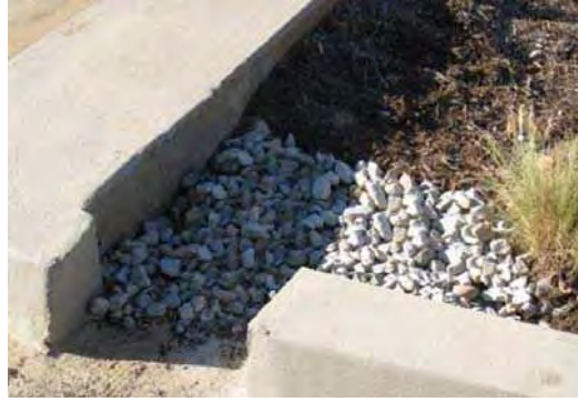
Figure 2: Curb Cut located in a Bioretention Facility
