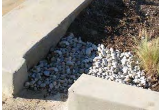
Figure 2: Curb Cut located in a Bioretention Facility
