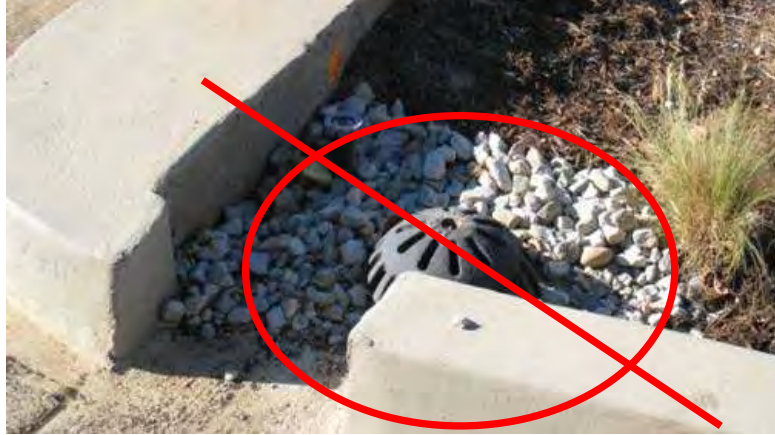
Figure 6: Incorrect Placement of an Overflow Inlet.
