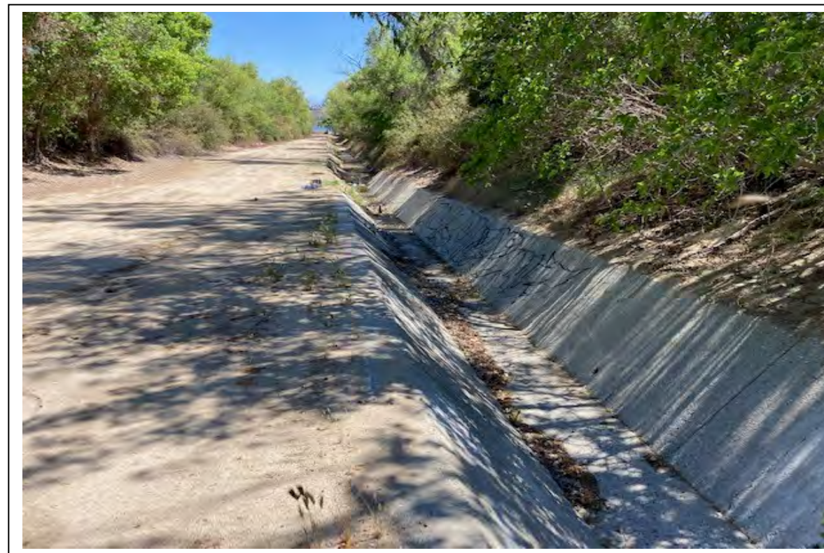
Photograph 6: June 2021. View depicting concrete portion of Hill Street Channel looking downstream towards Lake Elsinore. Note the transition to earthen channel in background.
