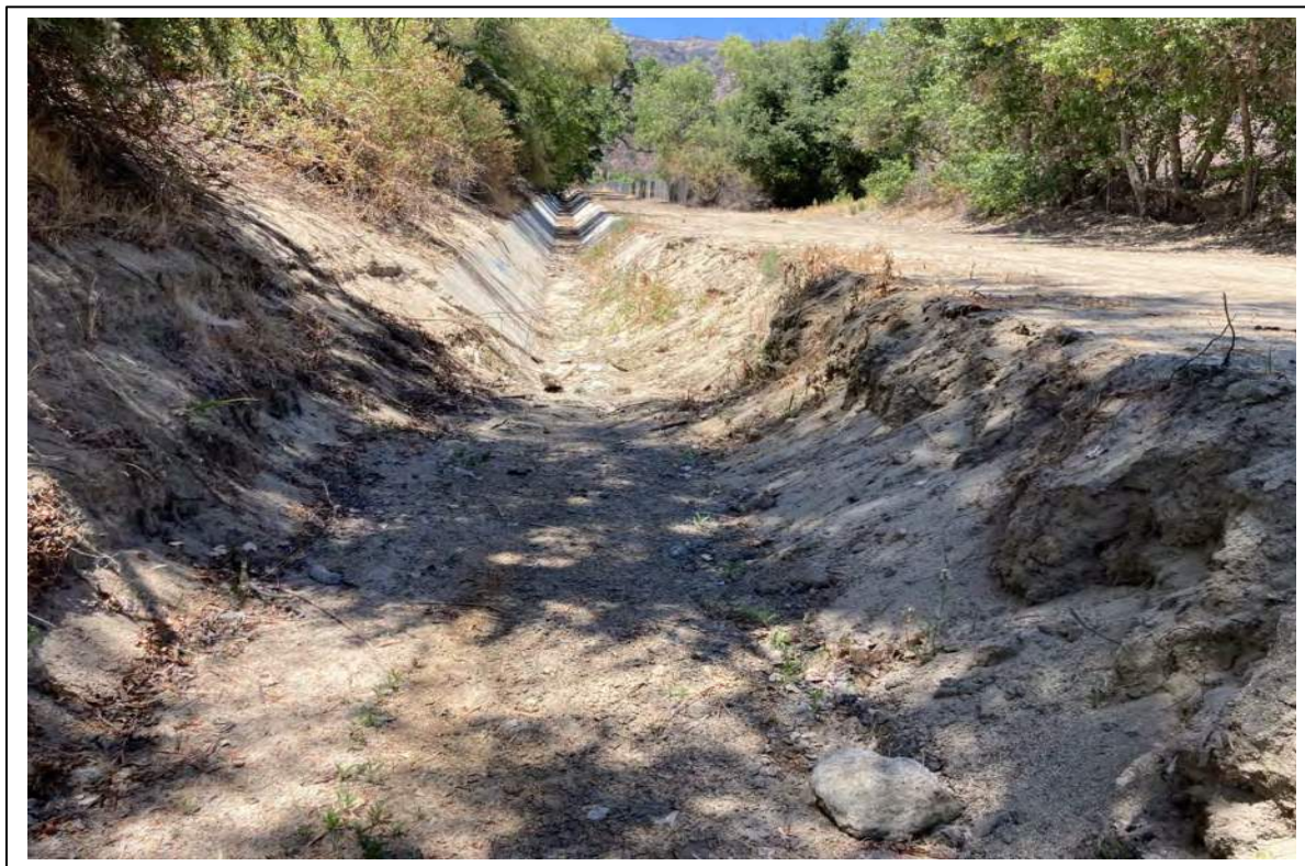
Photograph 7: June 2021. View of eroded earthen portion of Hill Street Channel looking upstream at concrete transition.
