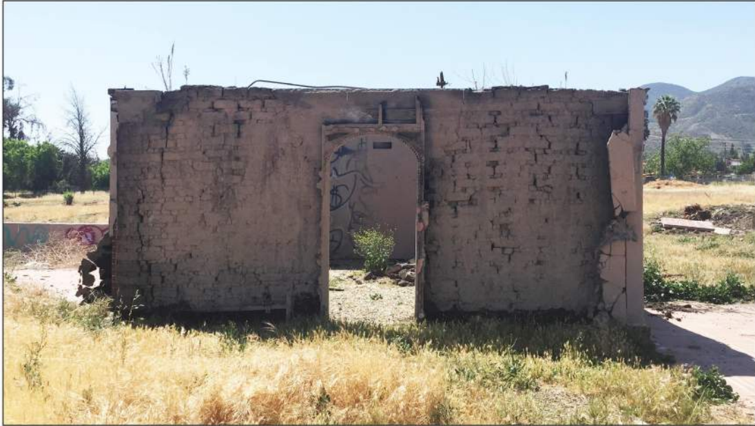
Plate 4.2-9: View of the non-original arched doorway in the north façade of the Machado Adobe, facing southwest. Note the framing around the doorway, indicating that the opening may once have been rectangular.
