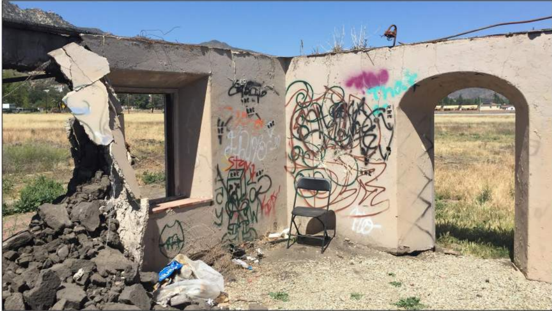
Plate 4.2–15: Interior view of the angled window and door jambs, facing northwest. The arched doorway is not original to the Machado Adobe.
