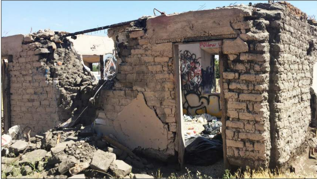
Plate 4.2-19: View of the west and south façades of the Machado Adobe showing the extensive damage to the building, facing north. Note the eroding of the adobe bricks at the base of the building due to water and fire damage.
