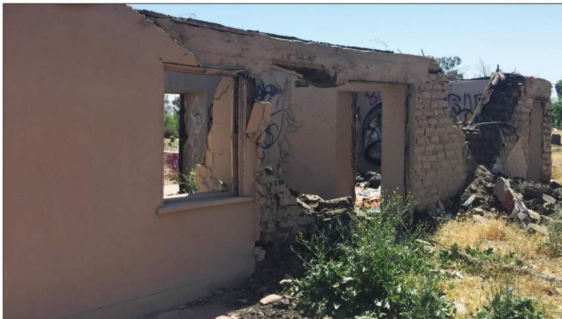
Plate 4.2-13: View of the crumbling stucco and adobe bricks on the west façade of the Machado Adobe, facing south. Note that portions of the wall have almost completely collapsed.
