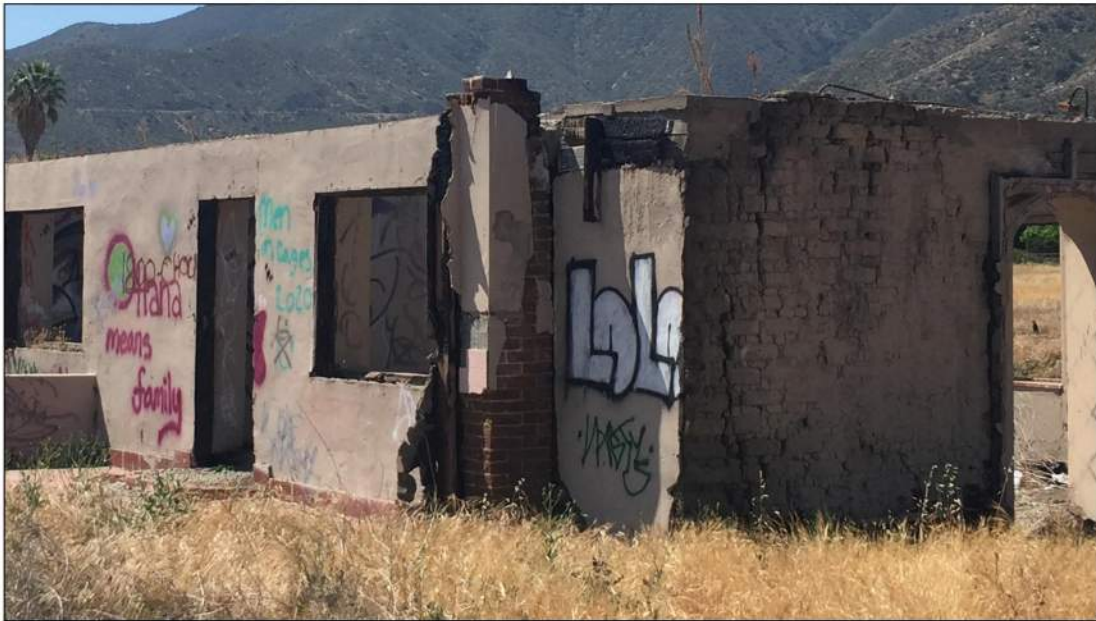
Plate 4.2–18: View of the likely non-original brick chimney located on the east façade of the Machado Adobe, facing southwest. Note the crumbling adobe bricks on the north façade (right).
