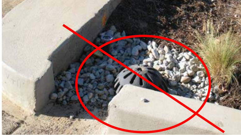
Figure 6: Incorrect Placement of an Overflow Inlet.
