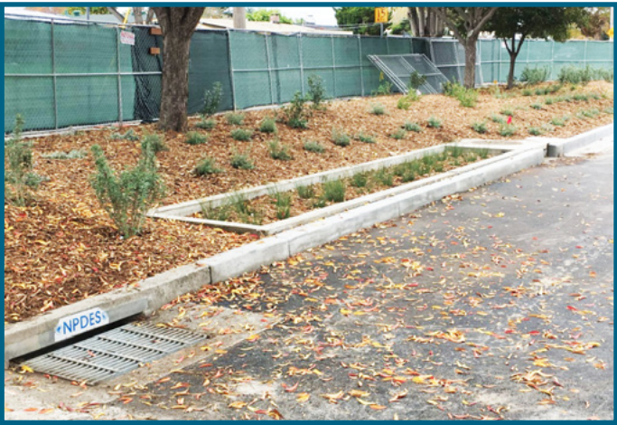
All-in-one treatment train, no need for separate trash capture manhole or vault.
