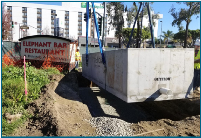
Simple vault and media installation.
