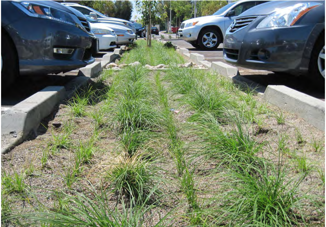
Figure A.9-1. Vegetated swale.
