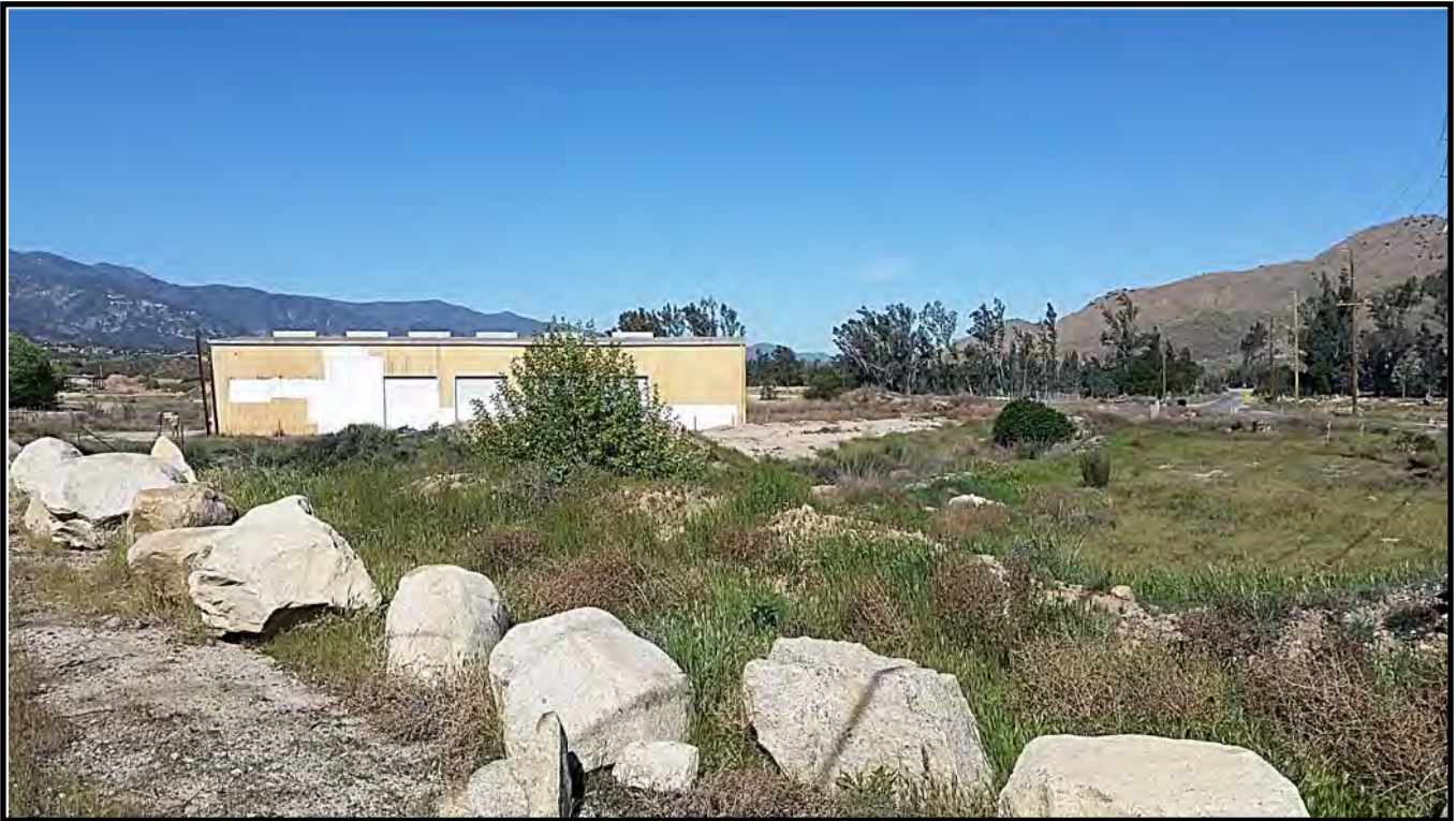
Looking west along the proposed Temescal Canyon Road realignment (The realignment will require the existing storage building be demolished)
