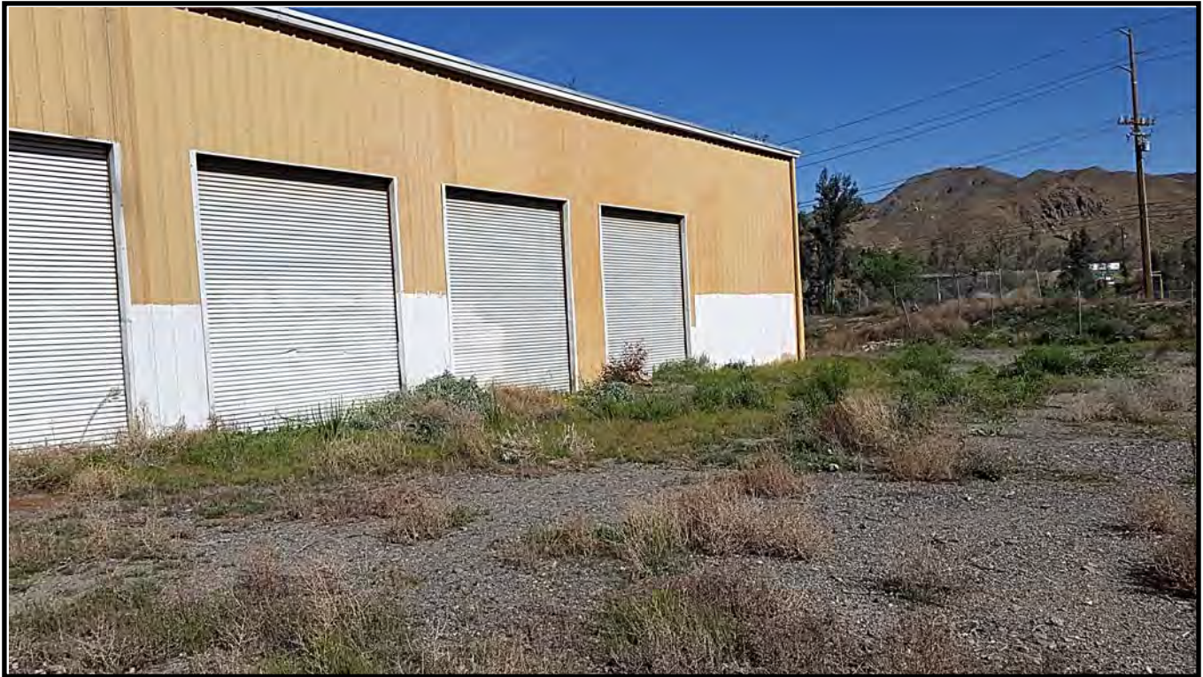
Looking north; The existing storage building to be demolished
