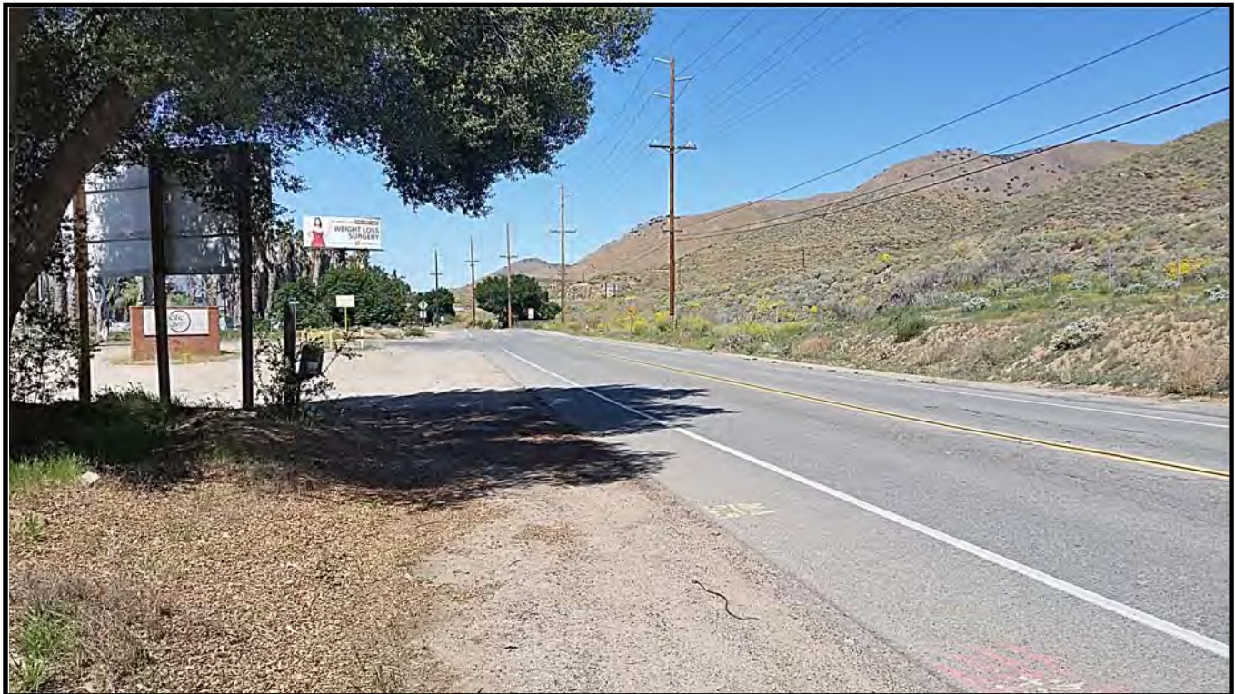
Looking west along the existing Temescal Canyon Road near Bernard Street, where the proposed realignment begins
