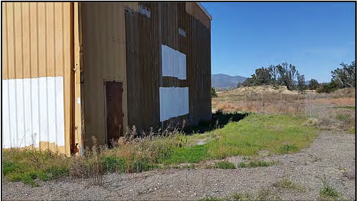
Looking west along north side of the storage building
