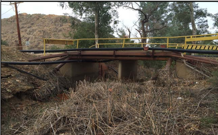
PHOTO #7: Bernard Street Bridge at Temescal Wash
