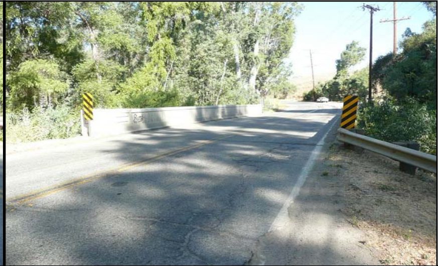
PHOTO #10: Existing Temescal Canyon Road Bridge looking west
