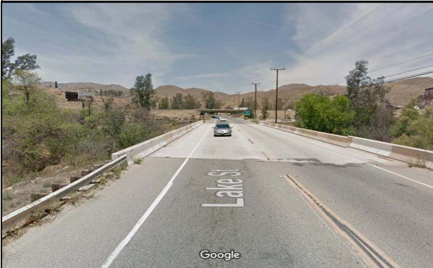
PHOTO #11: Lake Street Bridge looking north (Image taken from Google Earth)
