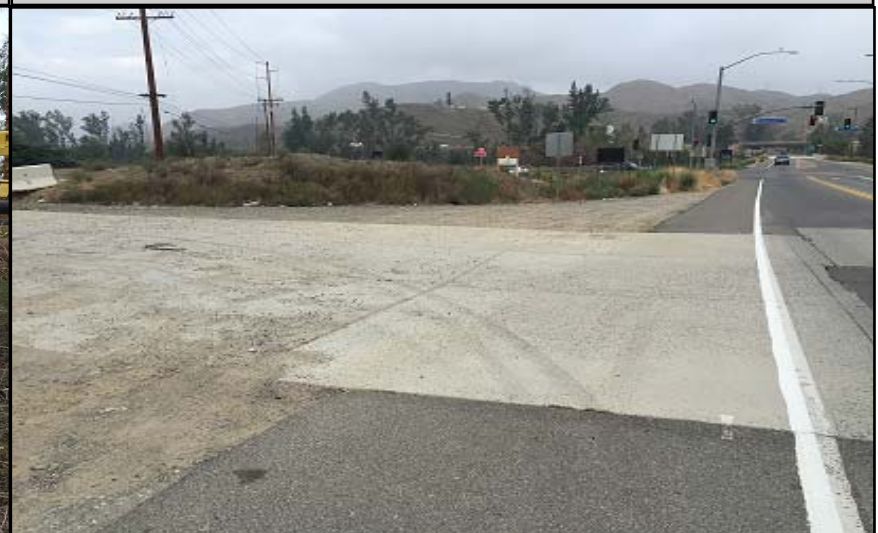
PHOTO #8: Lake Street looking north at location of the proposed tie-in of Temescal Canyon Road
