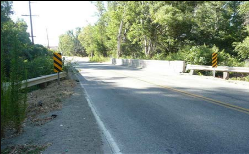
PHOTO #9: Existing Temescal Canyon Road Bridge looking east
