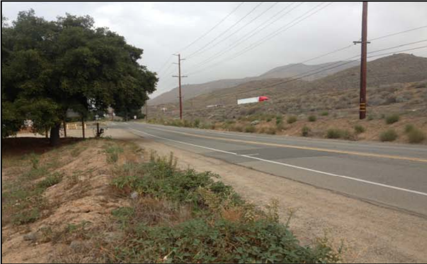
PHOTO #1: Looking westerly at the Existing Temescal Canyon Road near Bernard St.
