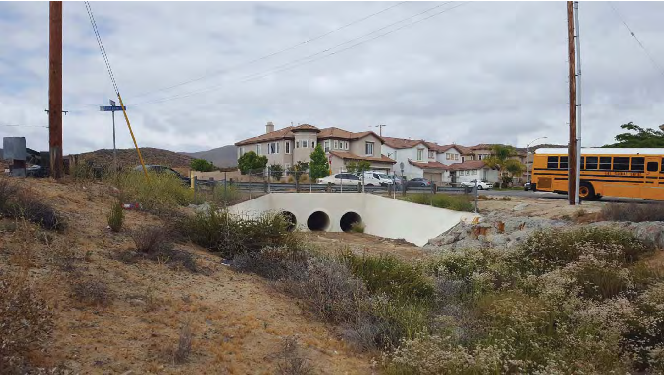
Existing Triple RCP Culvert at Canyon Estates Drive and Canyon View Drive
