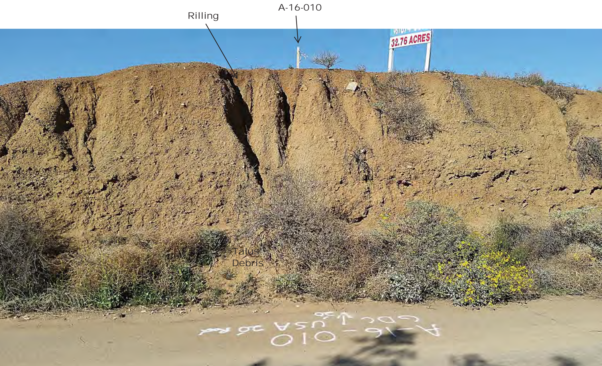
Existing Cut Exposing Alluvial Fan Deposits (Qyf) at A-16-010 Location
