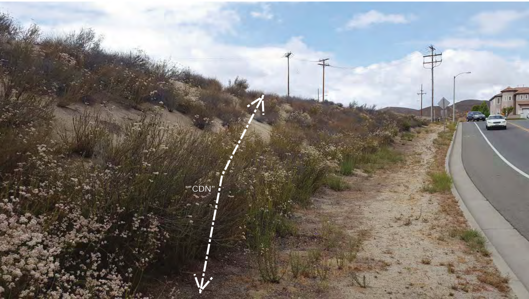
Existing Decomposed Granite Cut Slope along West Side of Canyon Estates to be Further Cut Into
