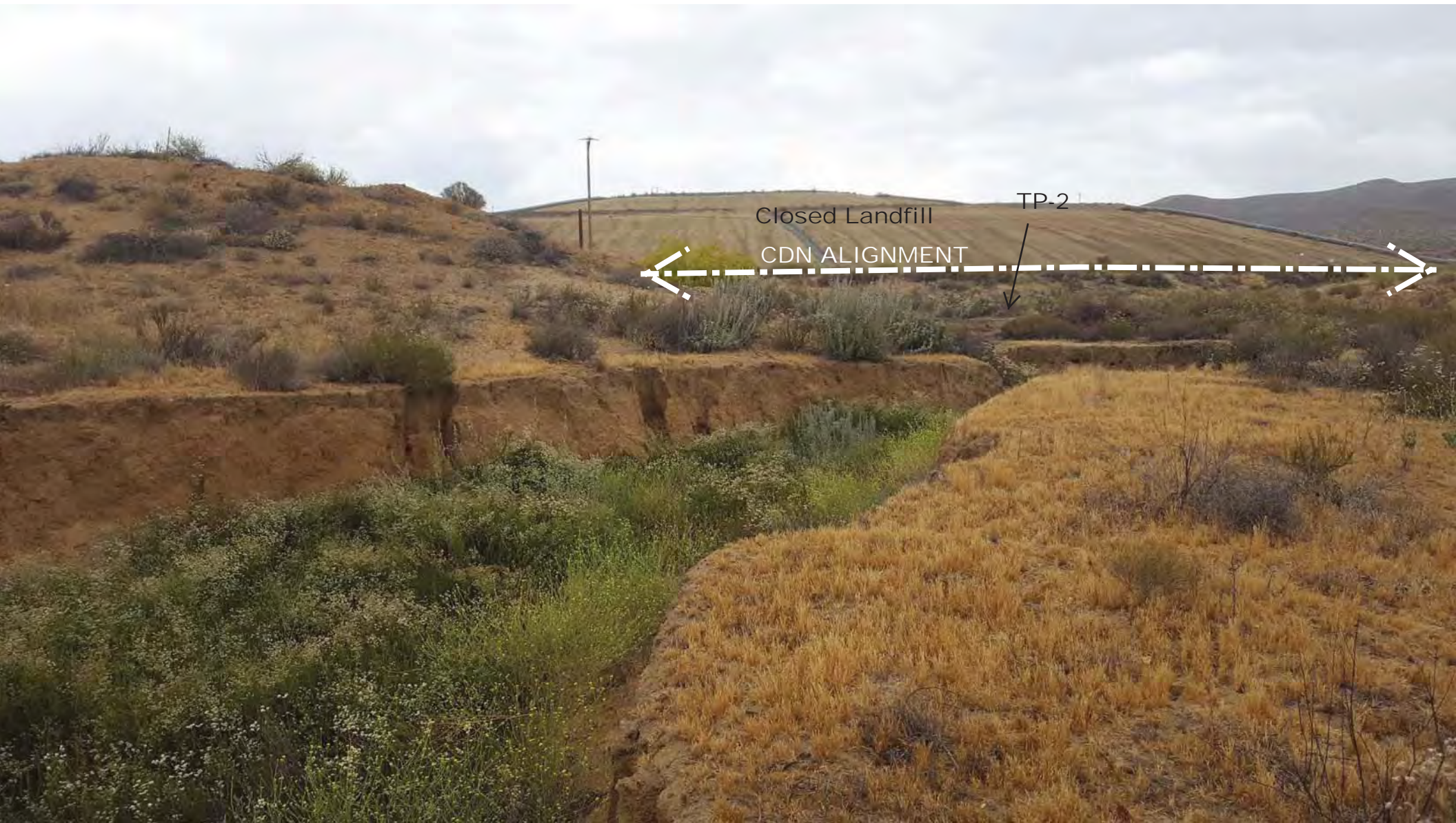
Eroded Gully Downstream of Station "CDN" 13+20
