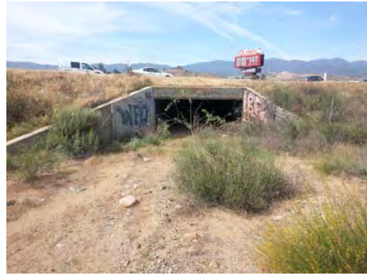
Photo 6 - 6'x14' Box Culvert at I-15 & Stovepipe Creek
