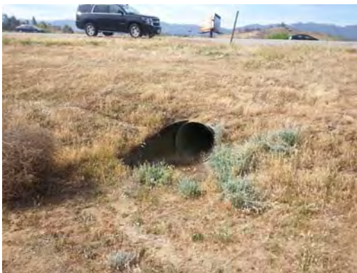
Photo 7 – 24" CMP along I-15 north of Stovepipe Creek
