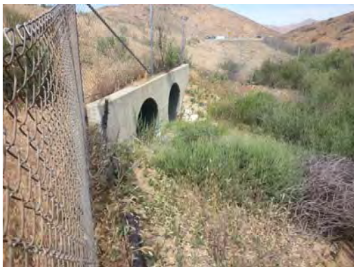
Photo 9 – two 48" RCP along I-15 North of Nichols Road.
