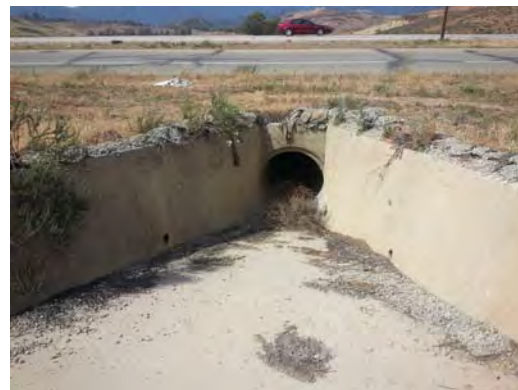
Photo 10 - 48" RCP along I-15 North of Nichols Road
