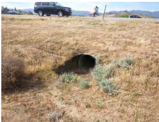
Photo 7 – 24" CMP along I-15 north of Stovepipe Creek
