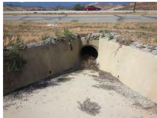
Photo 10 - 48" RCP along I-15 North of Nichols Road
