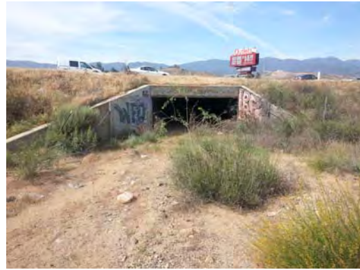
Photo 6 - 6'x14' Box Culvert at I-15 & Stovepipe Creek
