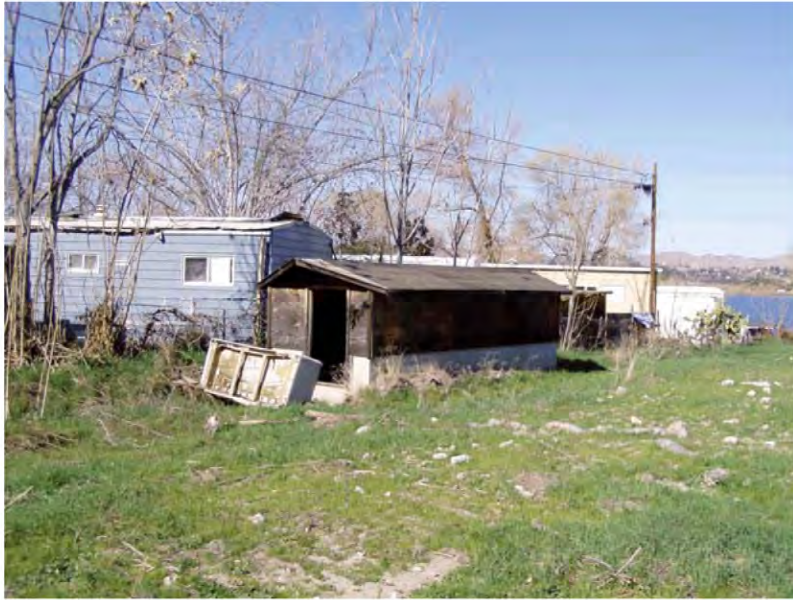
5. Northwest portion of site looking north. Note old sewer pump house onsite.
