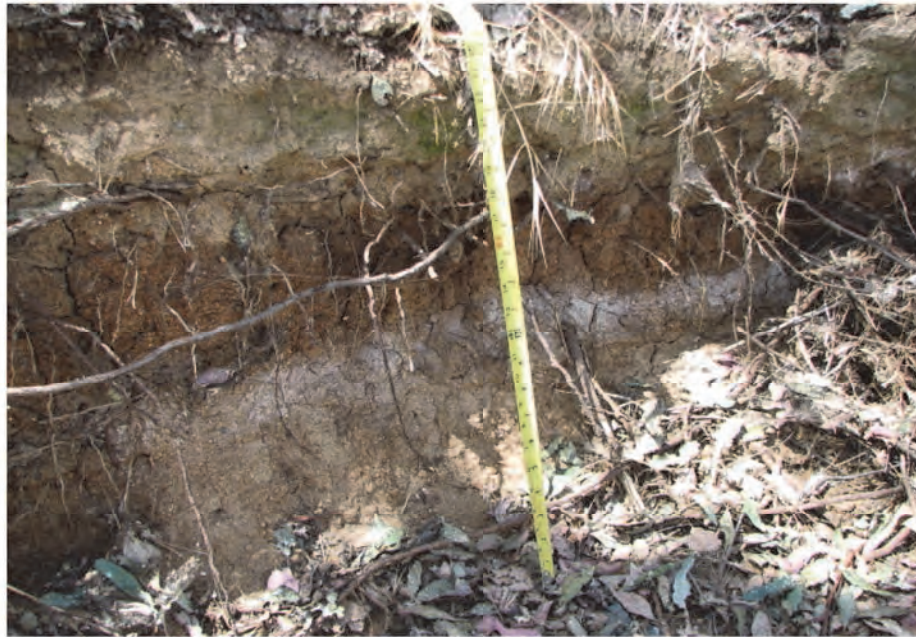
Photograph No. 5: Close up of erosional feature within trees
