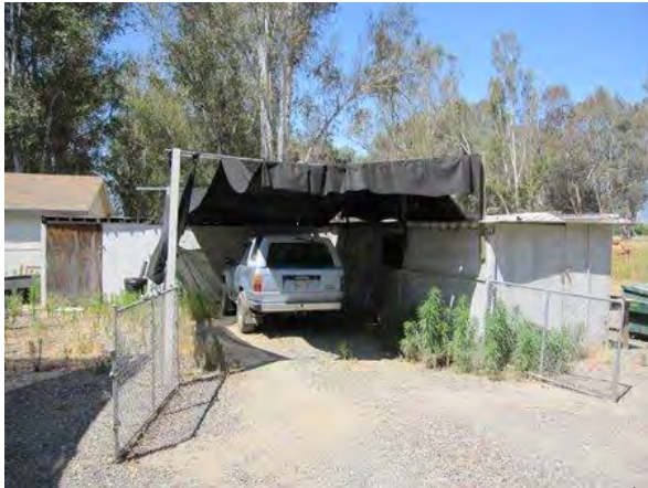
Photograph 5. View of storage shed at 29401 3 rd Street (looking southeast).
