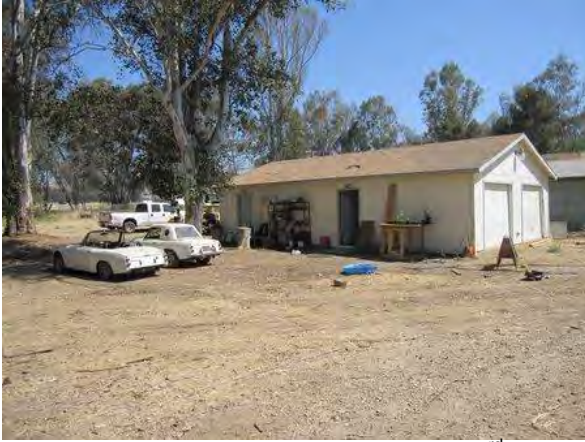
Photograph 9. View of garage at 29421 3 rd Street (looking north).
