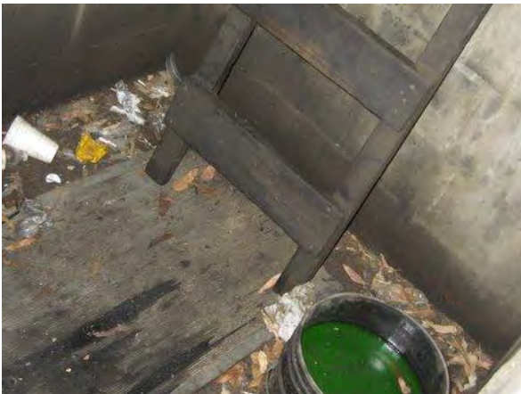
Photograph 13. Base of auto maintenance pit at 29445 3 rd Street. Pit is located below the car shown in Photograph 12.
