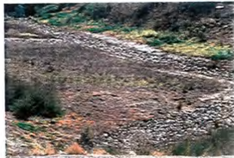
Figure 3: Gravel filled low-flow trench
