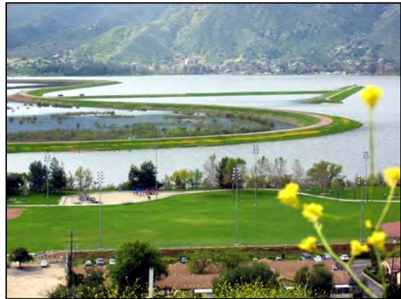
View of Lake Elsinore's Back Basin Levee
