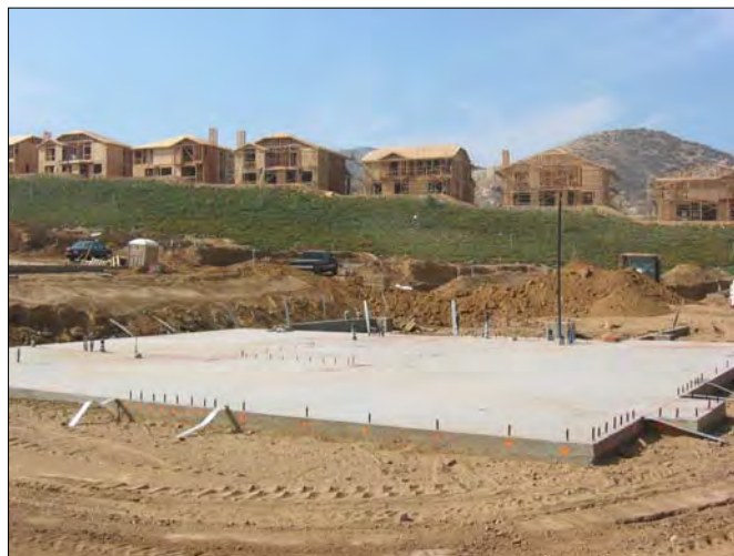
New tract home construction in City.
