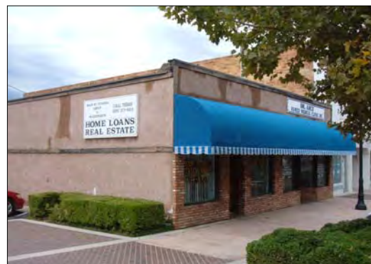
Historic building in downtown business district.
