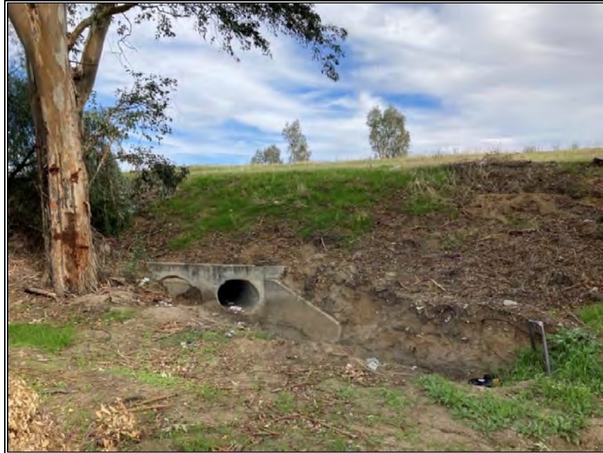
Photo 7. Two culverts, one of which is fully filled in with concrete, northeast of the Project site, facing north
